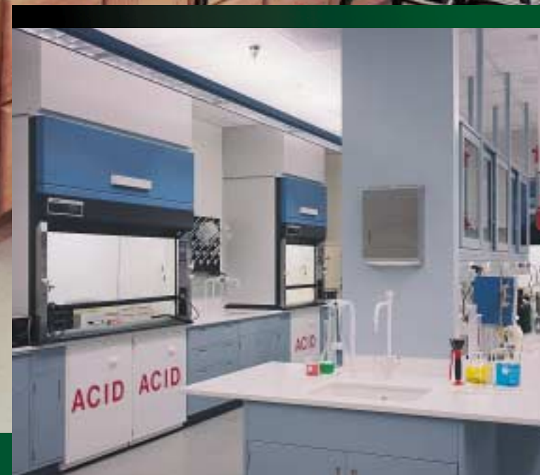
pale blue steel casework and white countertops. The hoods were customized with Phoenix Controls monitors and European-style service fixture fittings.
