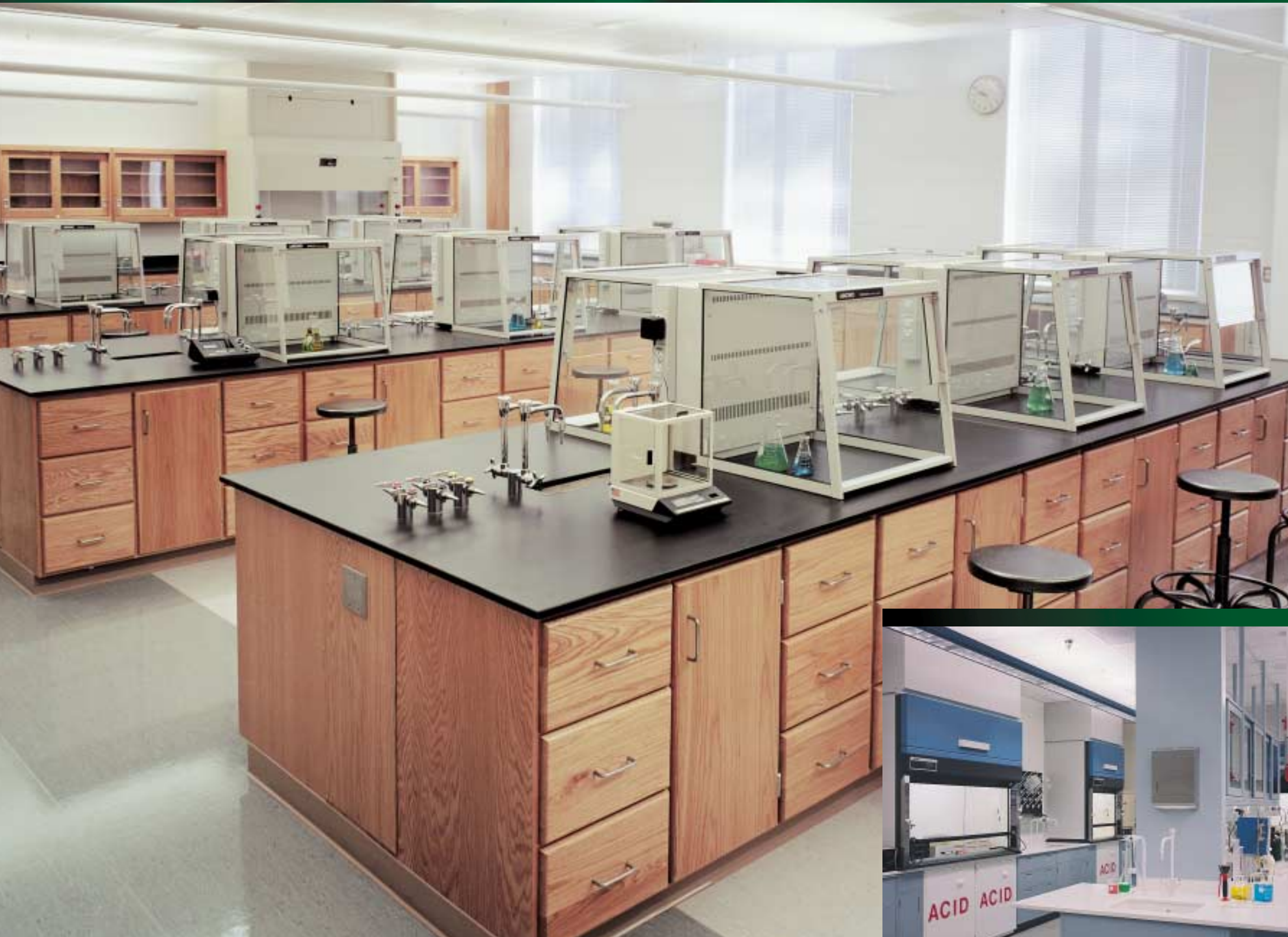
Above: Eighteen, two-foot Protector® VS Ventilation Stations fill this chemistry laboratory at Berry College, Mount Berry, Georgia. Glass sashes, sides and tops offer excellent visibility. In this unique installation, overhead ductwork was eliminated by ducting the Ventilation Stations through the casework, further enhancing visibility.
